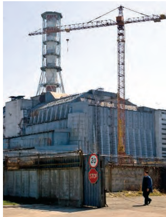
Sleeping giant. A guard walks past the remains of Chernobyl’s reactor #4, which is encased in a now-crumbling sarcophagus.
